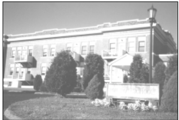
Pomeroy School reuse project Pittsfield, MA
