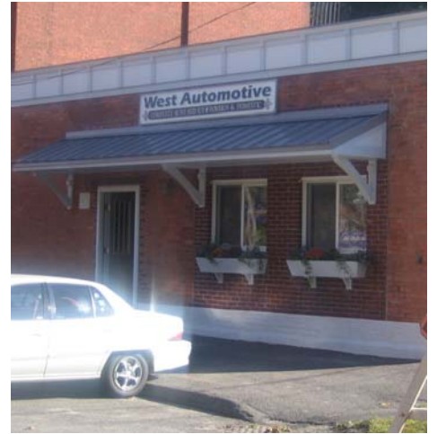
CDBG grant recipient West Automotive, pictured above, obtained a new sign and awning, brick repair and flower boxes.
