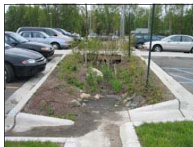
Bioretention Runoff Treatment Area in a Parking Lot
