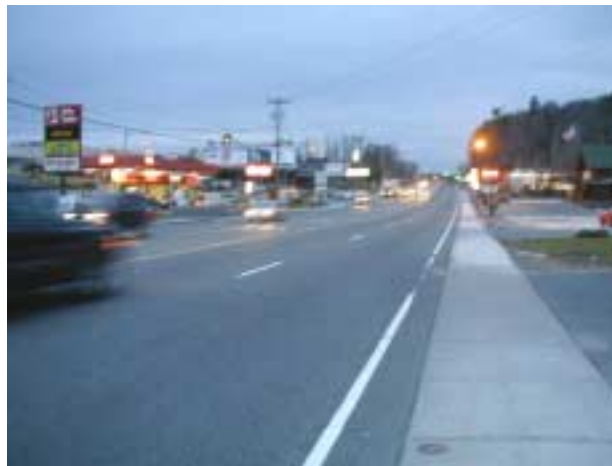
Photo 2: A rural road with frequent driveways on one side. Access management could be applied now before driveways are this dense all along it (Barker Rd., Pittsfield).
