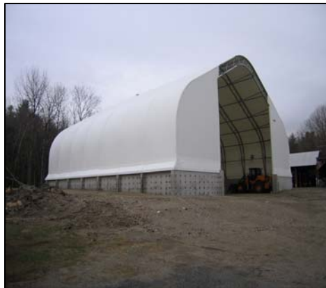
The Sandisfield Salt Shed
